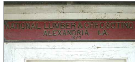
Originally incorporated as the National Lumber and Creosoting Company, the Alexandria, La., treating plant has been owned by Koppers, Roy O. Martin, Tangent Rail and others throughout its history.
